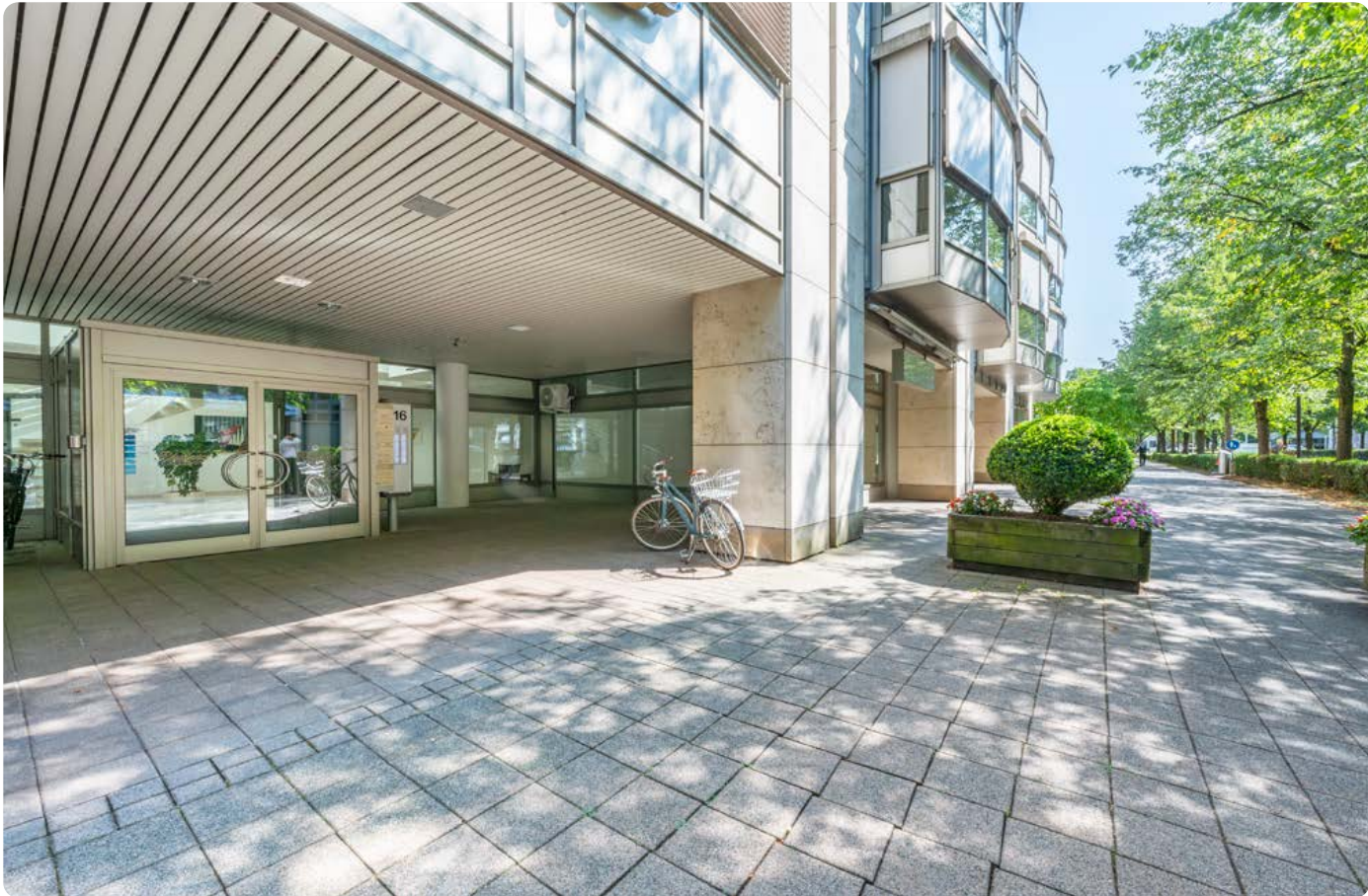
Covered entrance area
