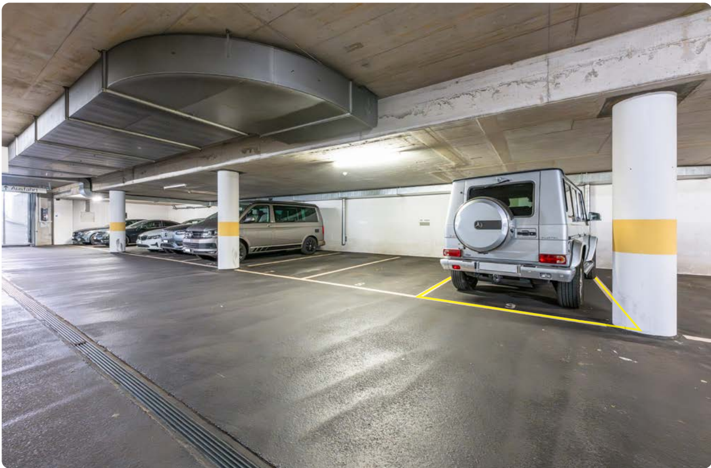
Underground parking space no. 9
