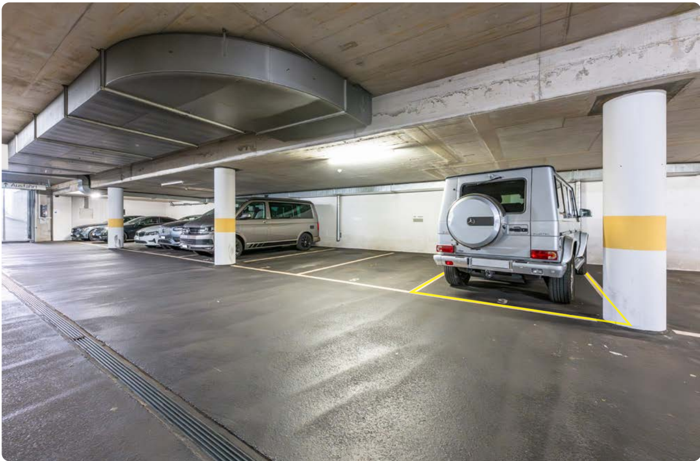
Underground garage no.9
