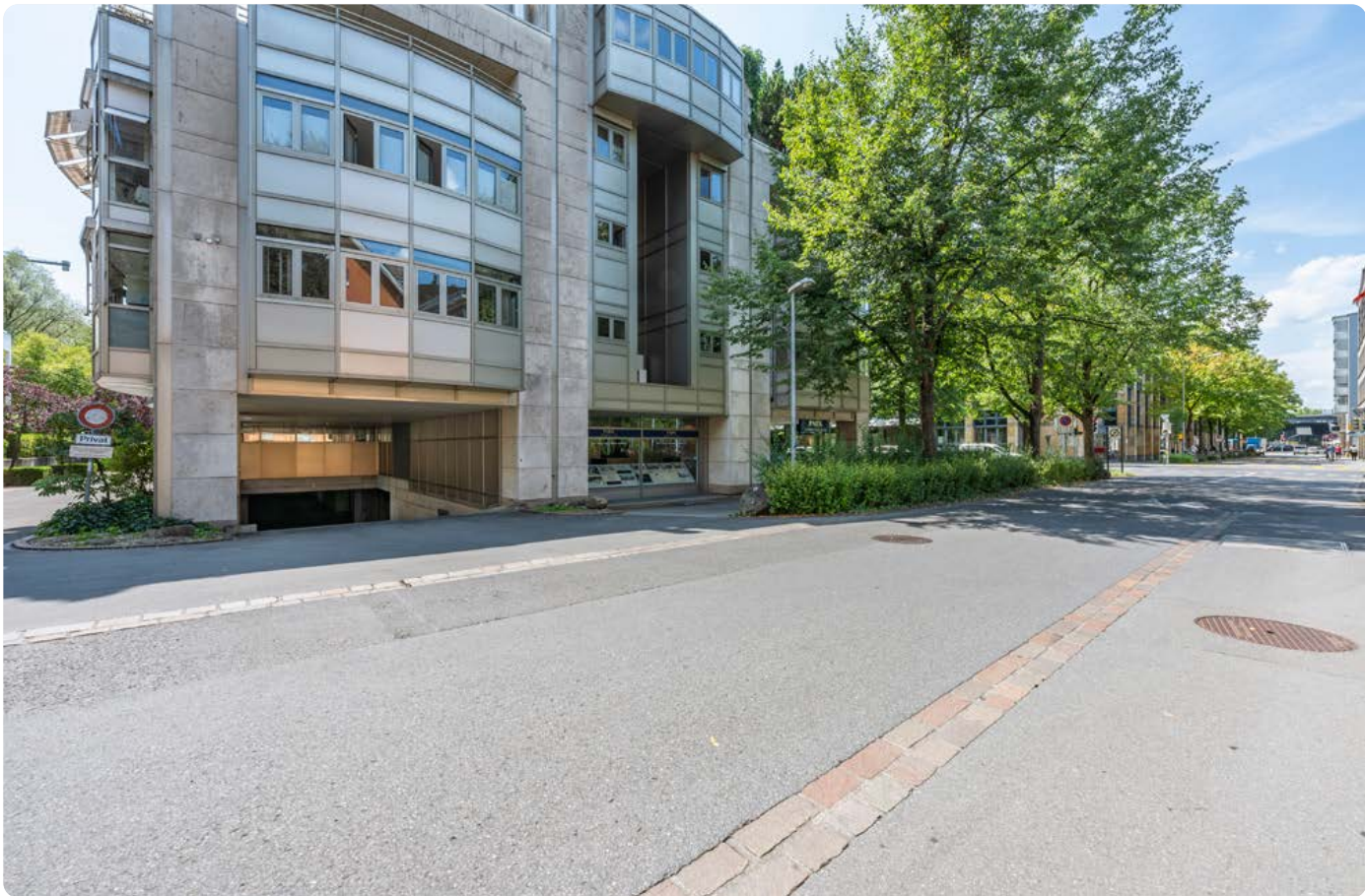
Underground garage entrance at Metallstrasse
