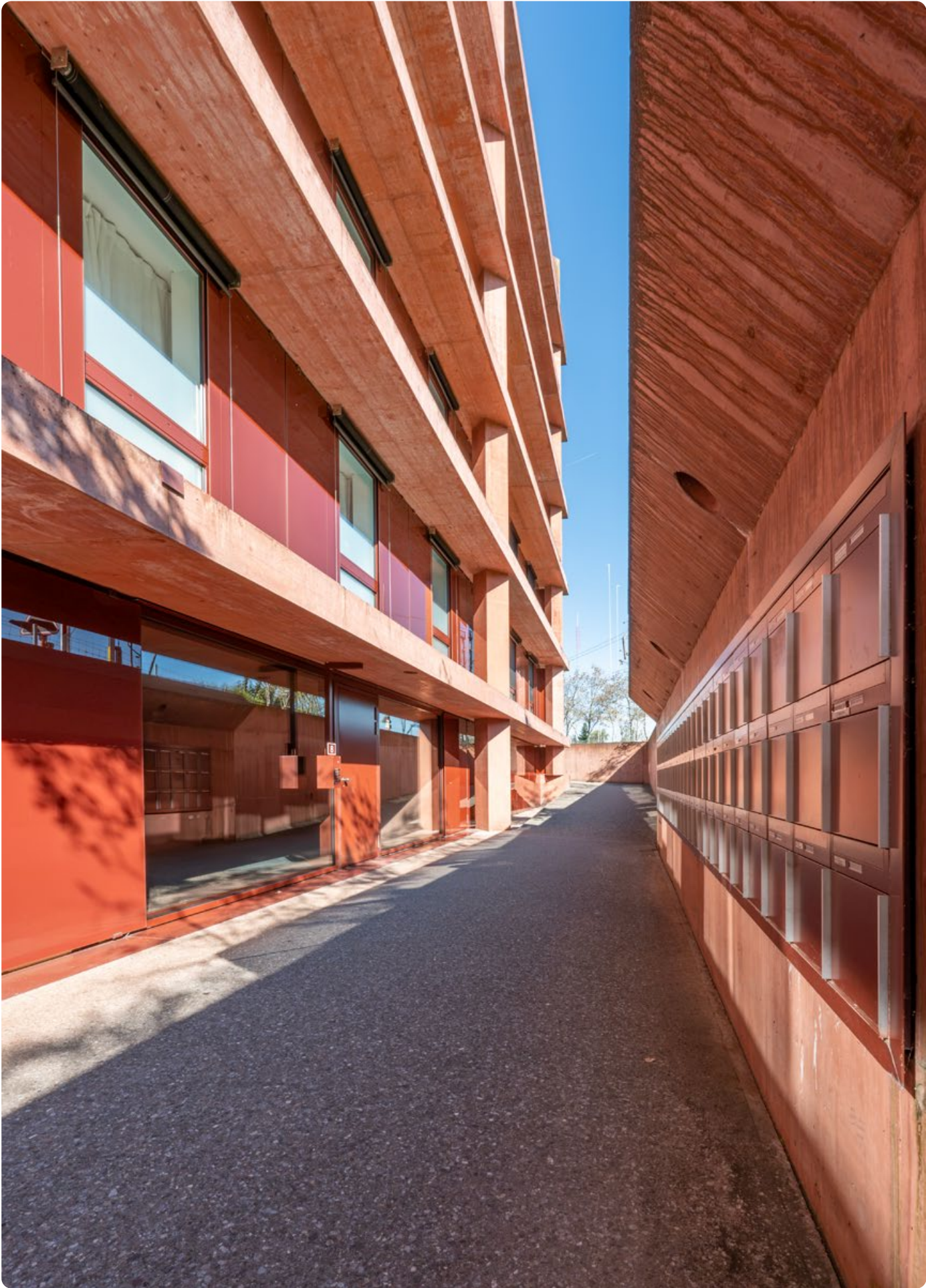
Architecturally designed entrance
