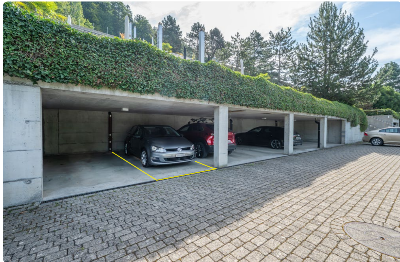
External parking space no. 14
