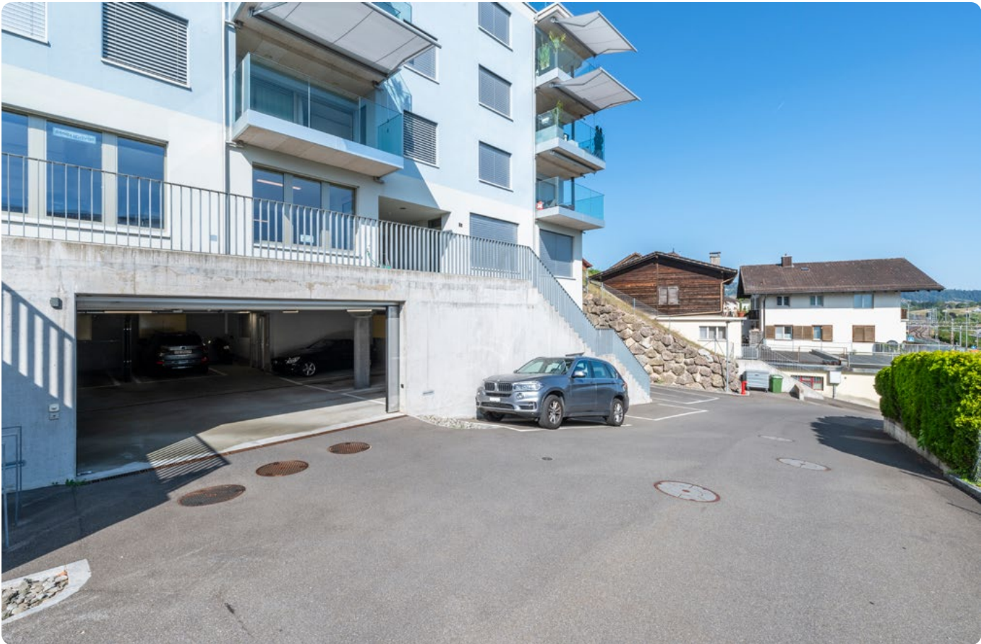
Underground garage entrance right next to the building
