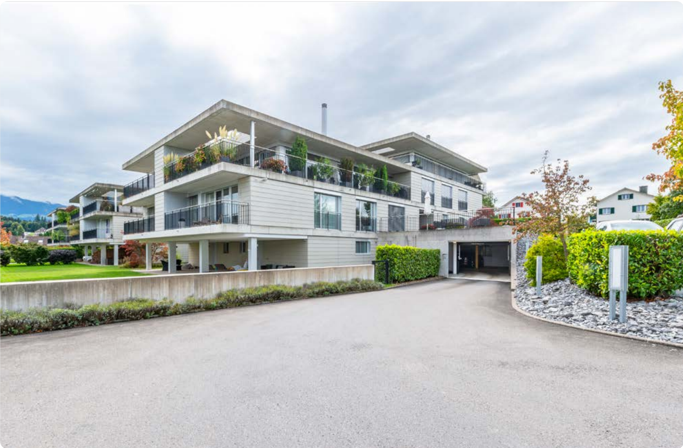
Underground garage entrance
