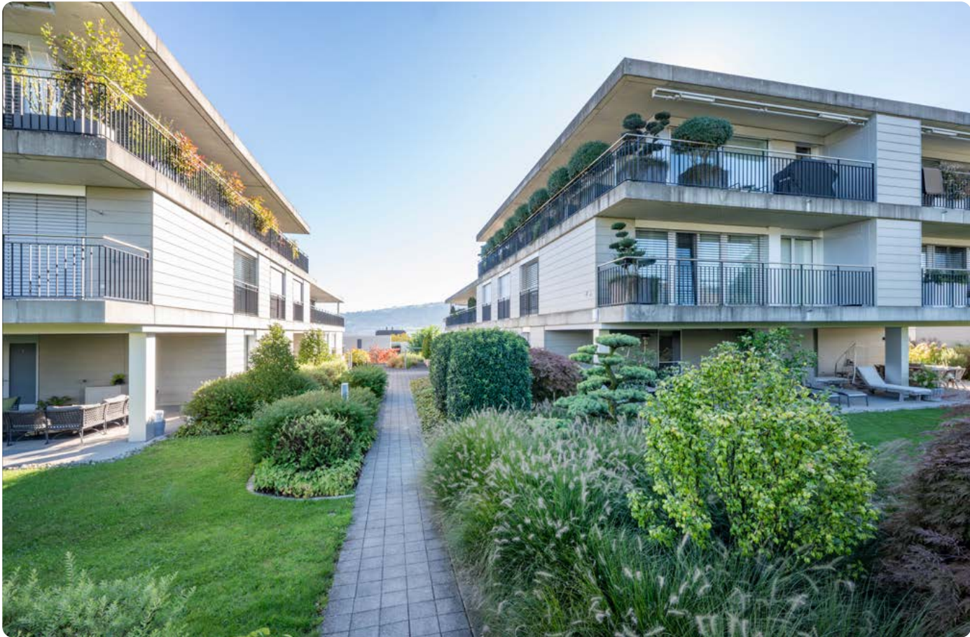
Access to the terraced houses
