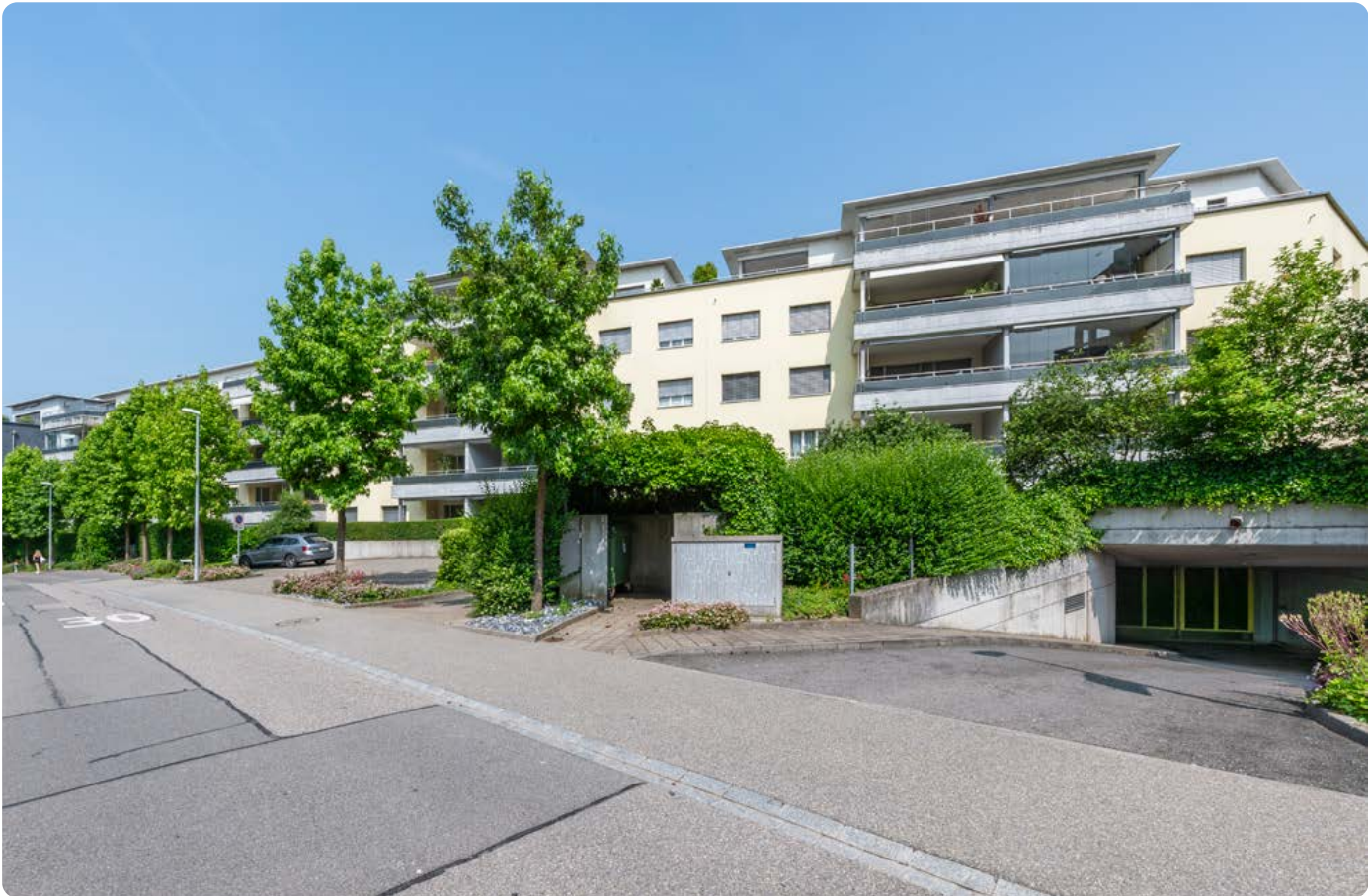
Underground garage entrance at Falkenweg
