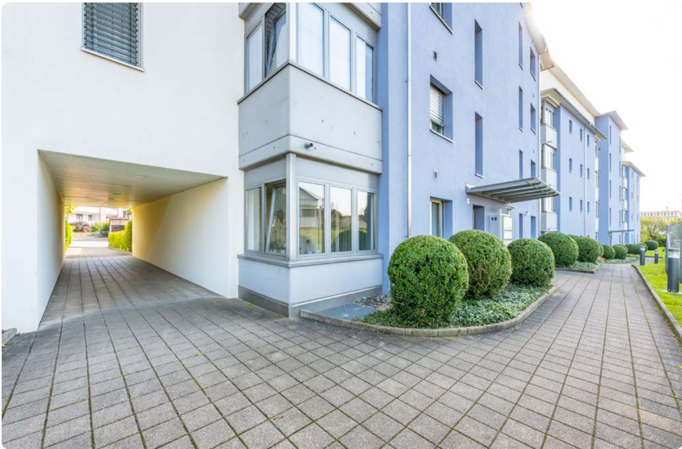
Main entrance on the north-facing side
