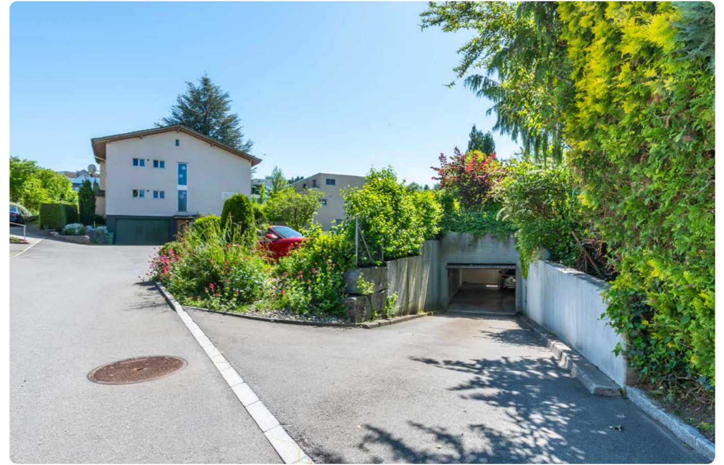
Underground garage entrance at Dorfring 18
